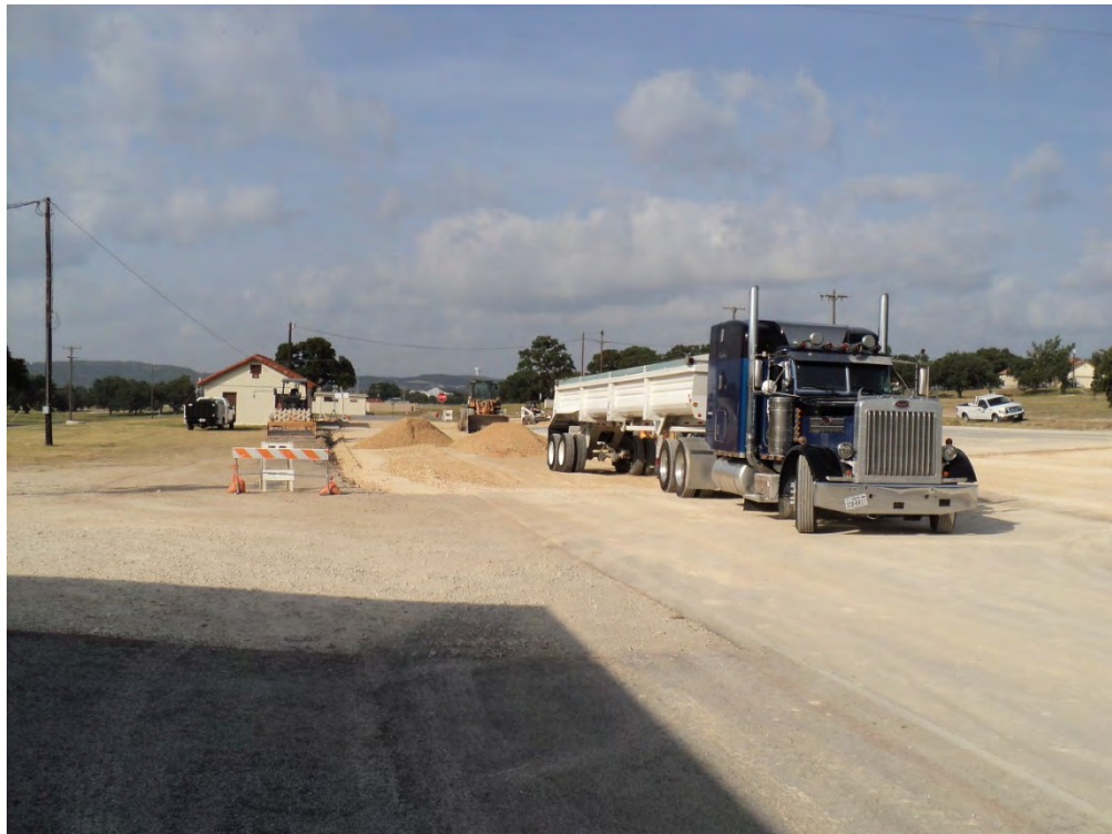
Photo 6. Placing base material (July 2013).
