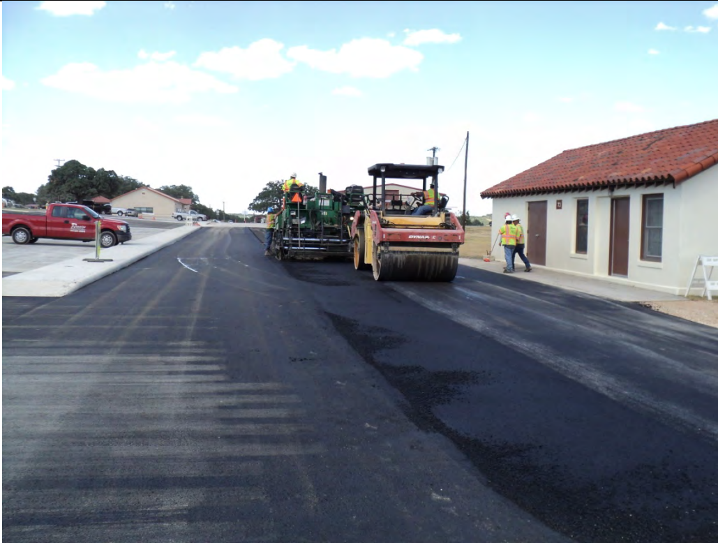
Photo 7. Paving the road in front of Building 73 (August 2013).
