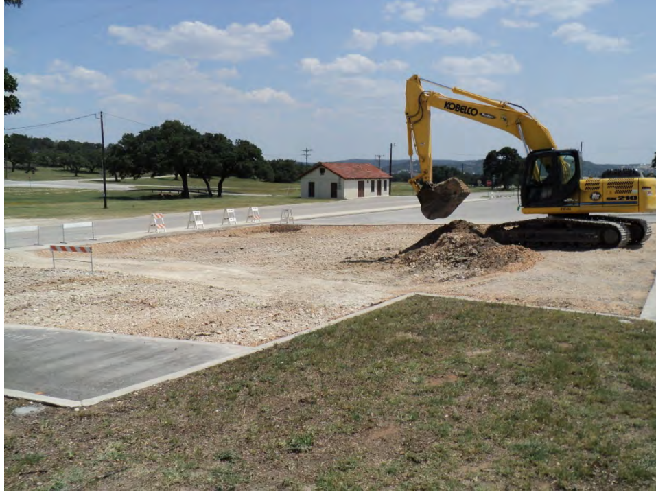
Photo 3. Excavating parking lot (July 2013).
