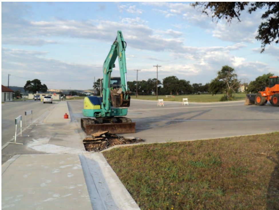
Photo 2. Initiating parking lot excavation (July 2013).
