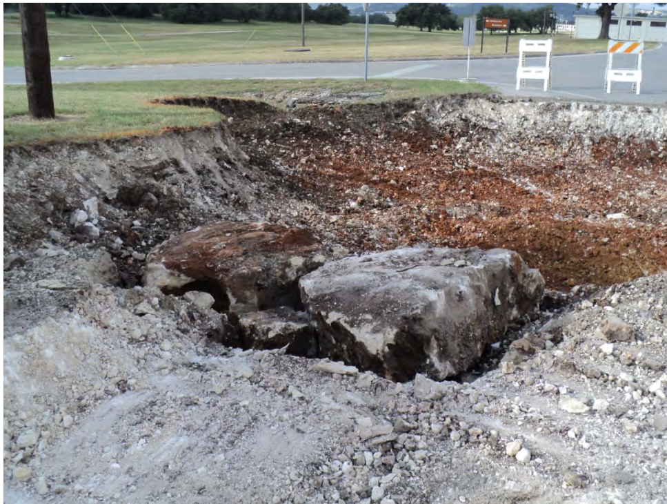
Photo 4. Excavating road area (July 2013).
