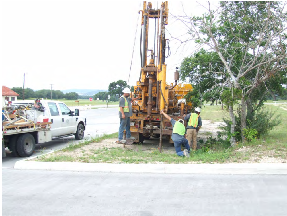
Photo 1. Parking Lot Investigation - drilling soil borings (June 2013).
