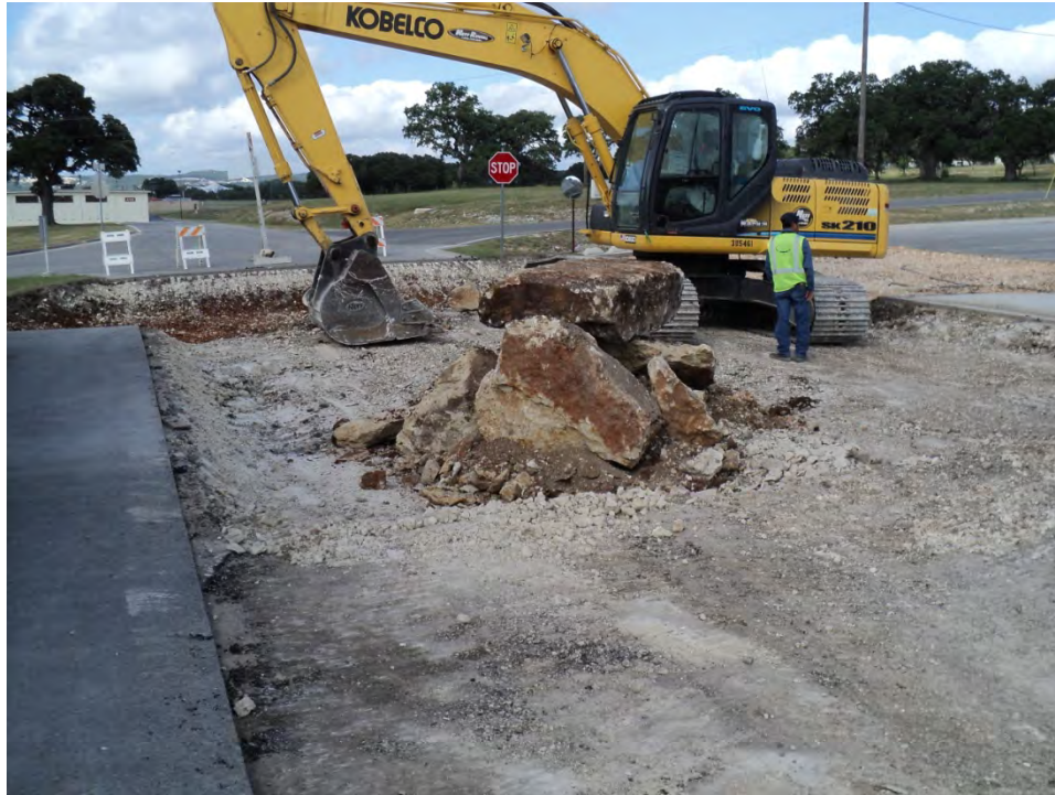
Photo 5. Large rock removed from excavation (July 2013).
