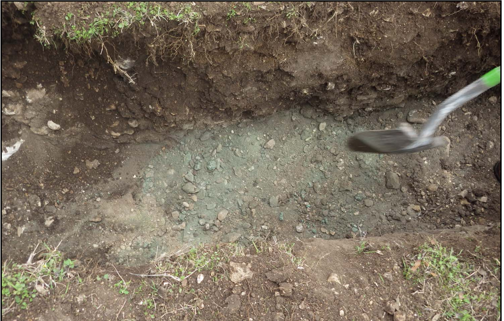
Photograph 1.1: Discolored soils discovered by a construction crew digging a trench to install a new fiber optic communication line. Approximate depth below ground surface is two feet.
