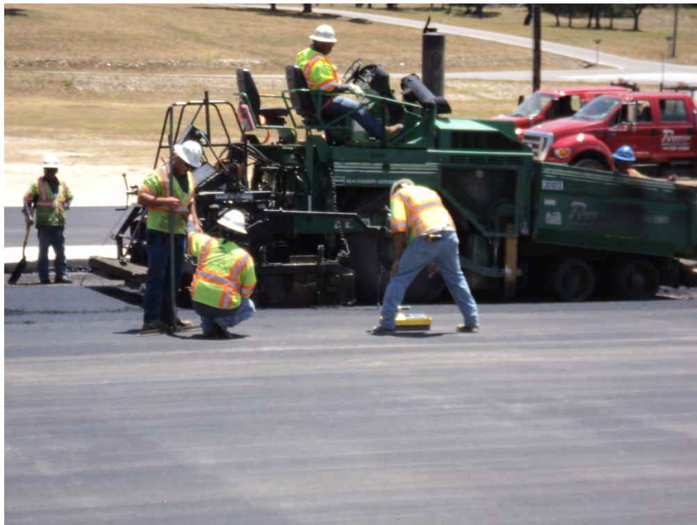
Photo 7. Density testing paved road (August 2013).
